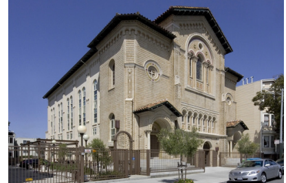
Photo Credit: Luke Thomas Photography for TNDC
